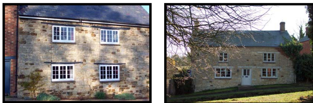
Photo 32 & 33 Traditional timber lintels
