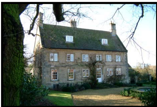
Photo 17 Wappenham House, faced in high quality ashlar masonry
