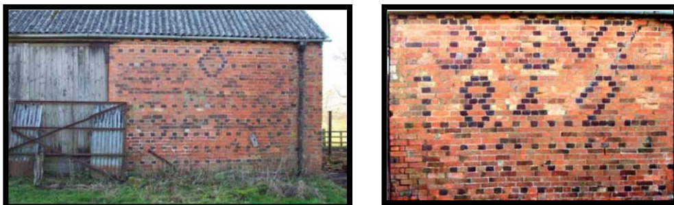
Photo 37 & 38 Brick Barn, with date and initials DM 1842
